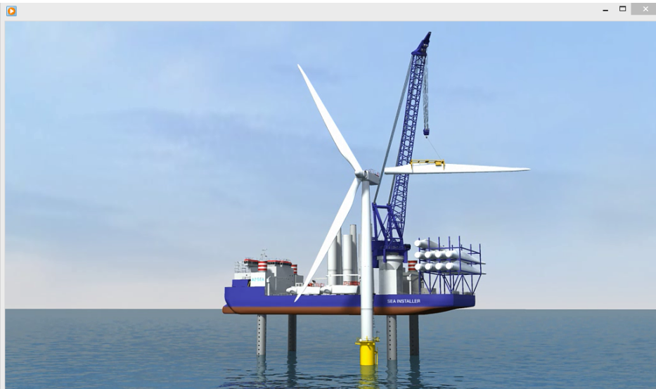
Borssele 01+02 Offshore Wind Farm
